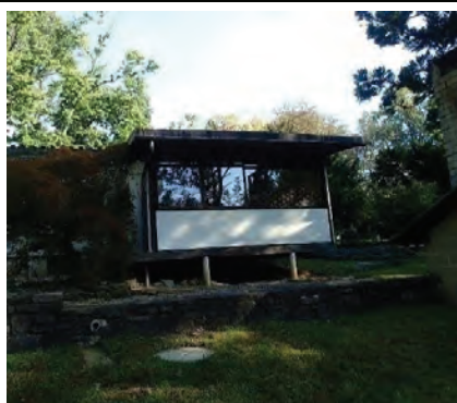
Fig. 2.8 1954 second build with partially open crawl space Photo credit: Michael C. Henry October 2023
