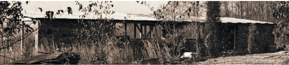
Figure 17.10 | A view of the north side of the house shows that the post-and-beam framework, along with the entire shed roof, both tile and corrugated sheet, were completed before the construction of the walls, ca. September 1947 (Source: Nakashima Foundation for Peace).
