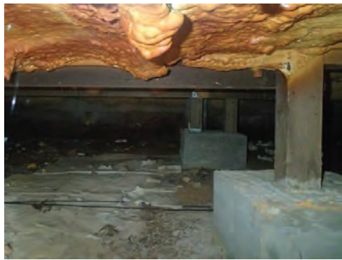
Fig. 2.53 SPF insulation & vapor barrier under 1946 build Photo credit: Michael C. Henry October 2023
