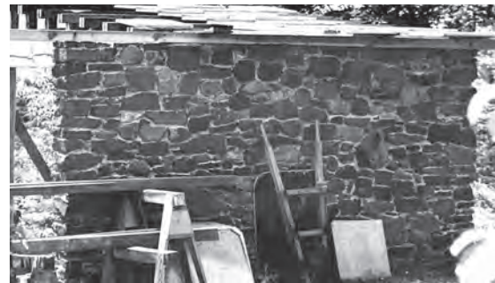
Figure 13.2 | A view looking southwest at the north stone elevation under construction. Constructed using irregular stones laid in anomalous pattern, this method is commonly known as uncoursed random rubble, ca. August 1947 (Source: Nakashima Foundation for Peace).
