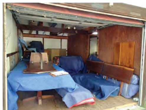
Fig. 2.56 Insulated interior of auto bay in the Garage Photo credit: Michael C. Henry October 2023
