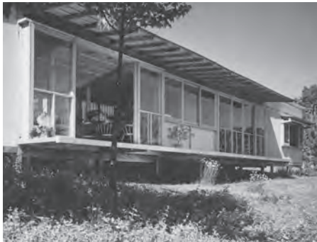
Figure 14.3 | The house after the first phase was complete. This view helps illustrate how elevated the house originally appeared, June 1949 (Source: Nakashima Foundation for Peace).
