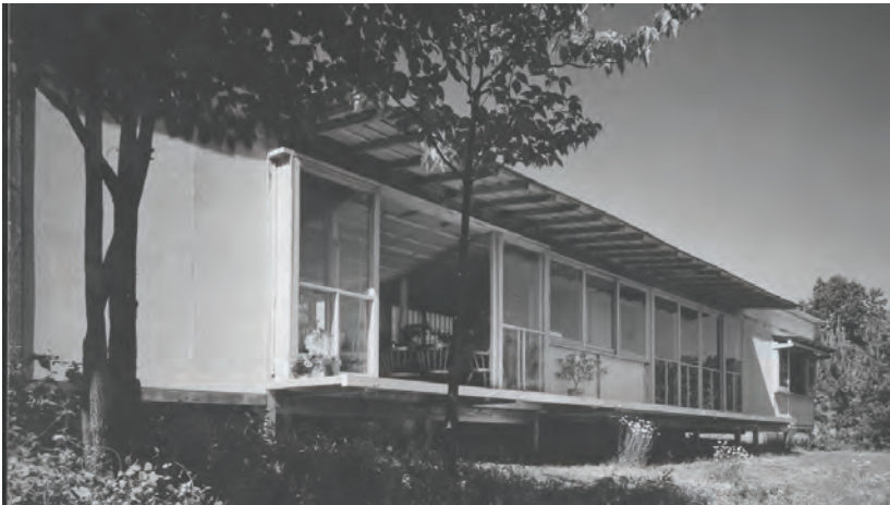
Figure 16.8 | A photograph taken after the construction shows how the original veranda dominated the south elevation, June 1949 (Source: Nakashima Foundation for Peace).
