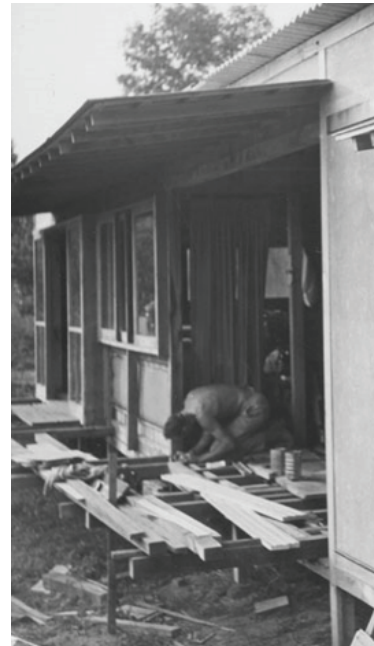
Figure 16.4 | This image partially shows the connection of the deck joists to the floor structure, providing some insight into how the deck was supported and integrated into the overall framework of the house, ca. September 1947 (Source: Nakashima Foundation for Peace).
