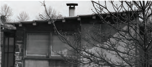
Figure 17.7 | view from the west shows the completed concrete tile construction, extending outward to create an awning over the window. This design not only provides shade but also helps protect the walls from rain, offering both functional and aesthetic benefits to the structure, ca. 1948 (Source: Nakashima Foundation for Peace).
