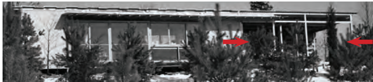
Figure 12.6 | The historic photo above it, taken sometime in the winter of 1946-47. It is used to emphasize that the west end of the building was fully enclosed, while the east side remained open, January 1948 (Source: Nakashima Foundation for Peace).
