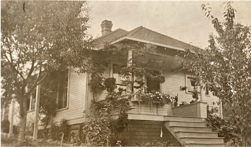
The "first" Nakashima family home. Located at 3808 South Genesee St., Seattle, the house stands on a corner lot with southern and western orientation. Note the pergola attachment on the west side to provide sun control and the lovely collection of plants on the porch. Photo, c. 1935, presumably taken around the time the family sold the house and moved to Portland, Oregon. (Michener Museum Archives; box 12, folder 26)
