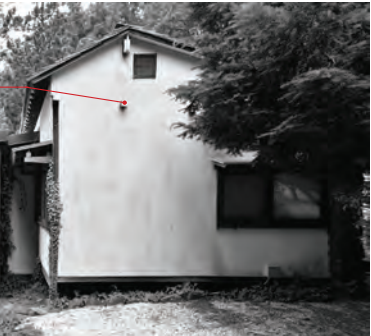
Figure 17.11 | East elevation of the Nakashima house with visible purlin supporting the original roof (Source: CAC, June 2024).
