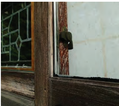
Fig. 2.12 Detail of window sash and insulated glass unit Photo credit: Michael C. Henry October 2023
