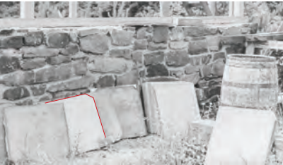
Figure 17.5 | A view of the house's initial construction from the northeast, looking toward the stone wall, shows the concrete tiles leaning against the wall. The chamfered corners of the tiles are visible as well, ca. August 1947 (Source: Nakashima Foundation for Peace).
