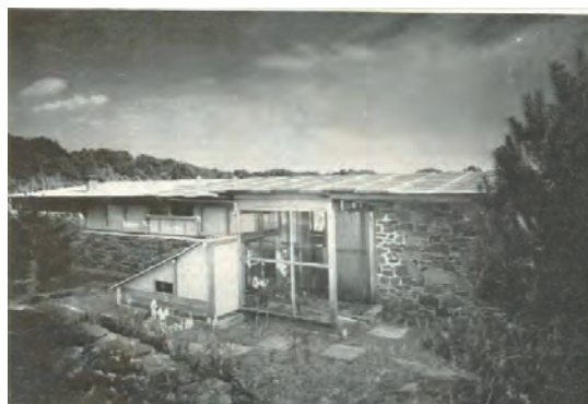
Fig. 2.5 Open-ended entry and two roofing materials Photo credit: Ezra Stoller No date
