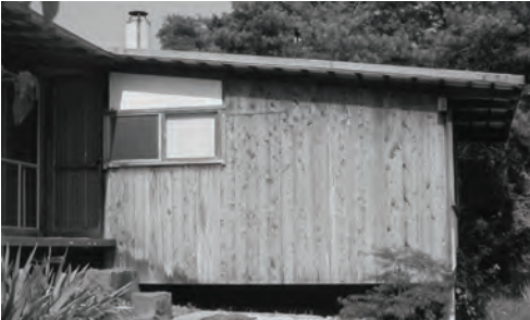
Figure 18.9 | A view looking toward Kevin's bedroom showing its original state, featuring wooden cladding on the west elevation, a chimney on top, and an exterior front door that opened onto the deck, July 1963 (Source: Nakashima Foundation of Peace).
