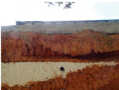
Fig. 2.55 SPF & polystyrene insulation under 1954 second build Photo credit: Michael C. Henry October 2023
