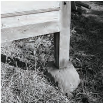
Figure 14.4 | A rubble stone plinth beneath the post at the exterior southeast corner of the parents' bedroom reveals the original Japanese pier-and-post foundation system, February 1952 (Source: Nakashima Foundation for Peace).
