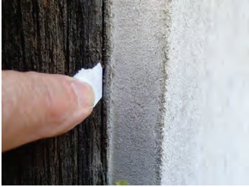
Fig. 2.10 Exposed edge of Cemesto Panel, SE corner, first build Photo credit: Michael C. Henry October 2023
