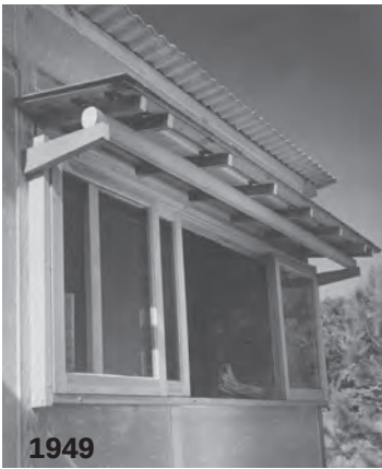
Figure 18.4 | Using the hyphen, Nakashima was able to retain the original four pane window on the south elevation of his own bedroom. While the addition blocked some of the window, his choice to extend out more than two feet ensured that the blockage would not significantly block the light (Source: Nakashima Foundation of Peace, June 1949 & CAC, June 2024).
