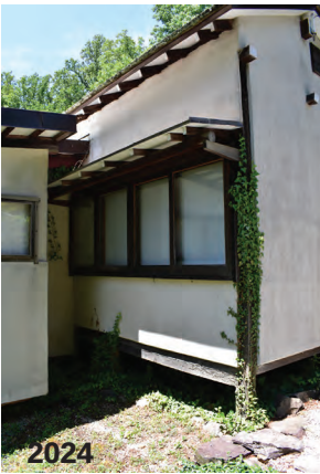
Figure 18.4 | Using the hyphen, Nakashima was able to retain the original four pane window on the south elevation of his own bedroom. While the addition blocked some of the window, his choice to extend out more than two feet ensured that the blockage would not significantly block the light (Source: Nakashima Foundation of Peace, June 1949 & CAC, June 2024).
