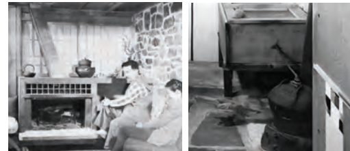
Figure 12.5 | A fireplace in the living room was the original primary source of heat in the house; however, a small coal burning water heater in the bathroom that provided hot water for the soaking tubs, may have offered additional warmth. Left: ca. 1948-56, Right: February 1952 (Source: Nakashima Foundation for Peace).
