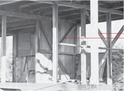
Figure 15.4 | A view looking southwest showing diagonal struts used in the walls around the bathroom, ca. September 1947 (Source: Nakashima Foundation for Peace).
