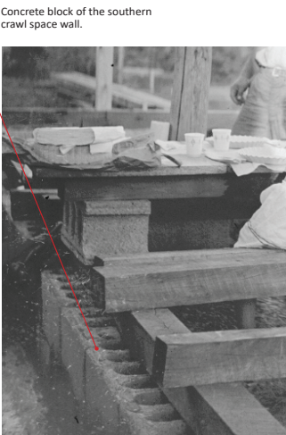
Figure 13.8 | A view looking east, showing the south block wall of the crawl space, as well as the chamber below the bathroom, ca. August 1947 (Source: Nakashima Foundation for Peace).
