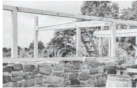
Figure 15.3 | A view looking southwest showing the primary girts running east-west and the transverse girts running north-south, ca. August 1947 (Source: Nakashima Foundation for Peace).
