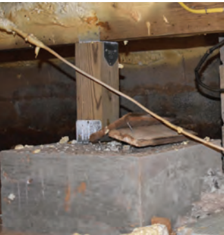
Figure 14.6 | A foundation post secured to the concrete footing using a metal plate (Source: CAC, June 2024).
