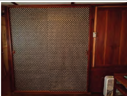
Fig. 2.18 Fabric-covered sliding door, main bedroom Photo credit: Michael C. Henry October 2023
