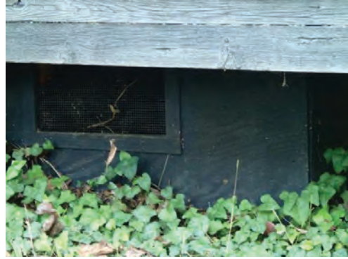
Fig. 2.52 Partial enclosure of crawl space, Parents' bedroom Photo credit: Michael C. Henry October 2023
