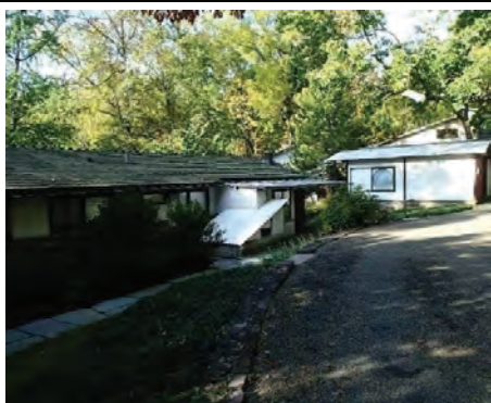
Fig. 2.6 1982 Third Build Roof, House set into brow of hill Photo credit: Michael C. Henry October 2023
