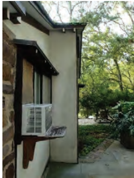
Fig. 2.39 Lack of gutter on north side of 1982 third build Photo credit: Michael C. Henry October 2023
