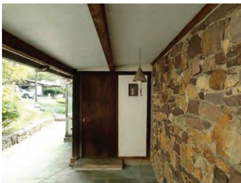
Fig. 2.4 Enclosed Entry Photo credit: Michael C. Henry October 2023
