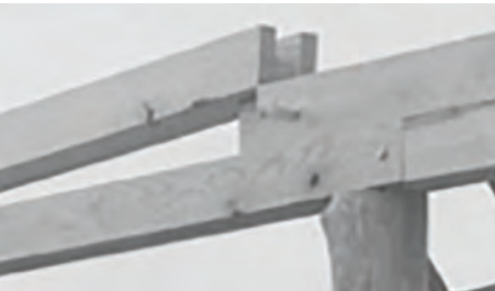
Figure 15.7 | Joint detail of transverse girts placed on the mother post, ca. August 1947 (Source: Nakashima Foundation for Peace).
