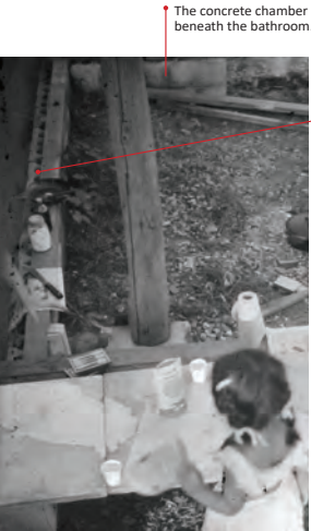
Figure 13.7 | A view looking east showing the south concrete block wall of the crawl space, as well as the chamber below the bathroom, ca. August 1947 (Source: Nakashima Foundation for Peace).
