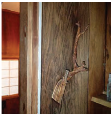
Fig. 2.16 Handle on interior door Photo credit: Michael C. Henry October 2023
