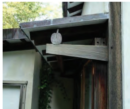
Fig. 2.13 Protective overhang at window Photo credit: Michael C. Henry October 2023
