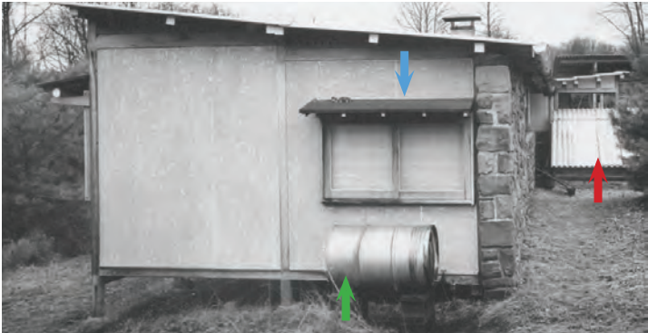
Figure 12.7 | A view looking west shows the presence of an additional chimney on the roof and a tank likely used for storing kerosene for new heating system, February 1952 (Source: Nakashima Foundation for Peace).
