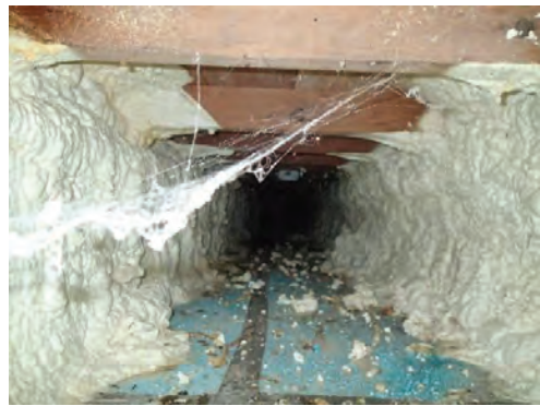
Fig. 2.54 SPF insulation in linear crawl space along north wall Photo credit: Michael C. Henry October 2023
