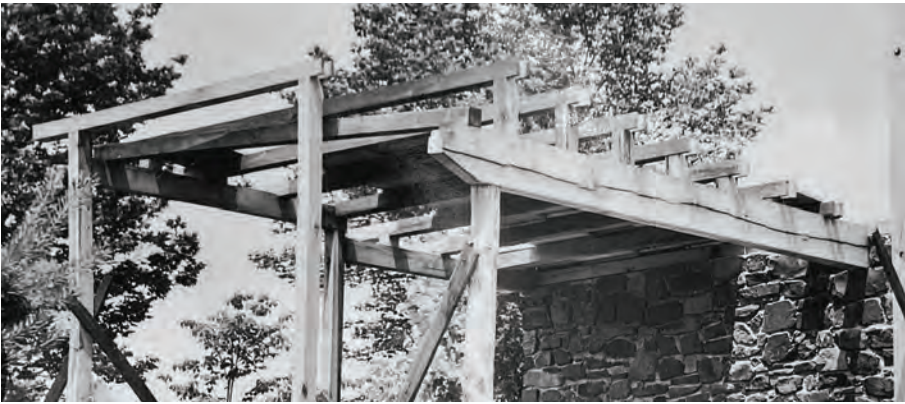
Figure 15.5 | A view looking west showing the small intermediate struts placed on top of the transverse girts ensuring the necessary slope for the roof purlins. Open mortises are visible and ready for connection to extend the purlins using tenon joinery, ca. August 1947 (Source: Nakashima Foundation for Peace).
