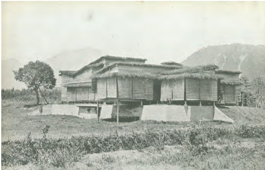
Raymond Summer Studio, view with Mt. Asama in distance, 1933. Thatch roof and “sudare”, or reed blinds, are traditional methods of heat control during summer. (AAUP, Raymond Col.)
