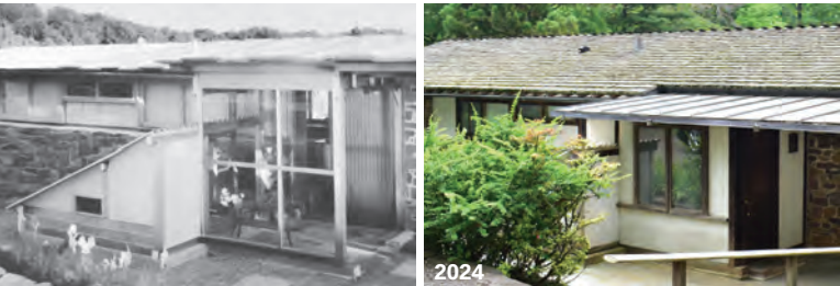
Figure 12.9 | The entry way into the house on the north elevation shows that it was much less closed in than it is today, with the entire west wall open and the north wall large open glass panels (Source: Nakashima Foundation for Peace, June 1949, and CAC, June 2024).
