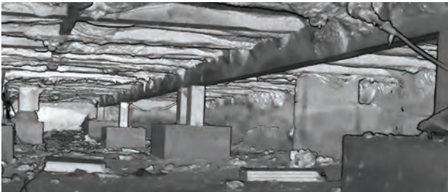
Figure 14.8 | Two images created from laser scan data reveal the complexity of the foundation area of the house including the major east-west, horizontal beams that are supported by the vertical struts, placed on top of concrete footings. The textured surface at the top of the images is the result of spray foam that was applied to the underside of the floor to improve insulation (Source: CAC, June 2024).
