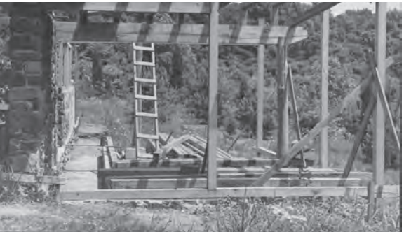
Figure 14.9 | A view looking east both the horizontal joists that run north/south, on top of the primary beams. In addition are several of the vertical struts that support the roof, ca. August 1947 (Source: Nakashima Foundation for Peace).
