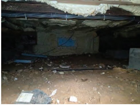
Fig. 2.51 Partial enclosure of crawl space under 1954 build Photo credit: Michael C. Henry October 2023
