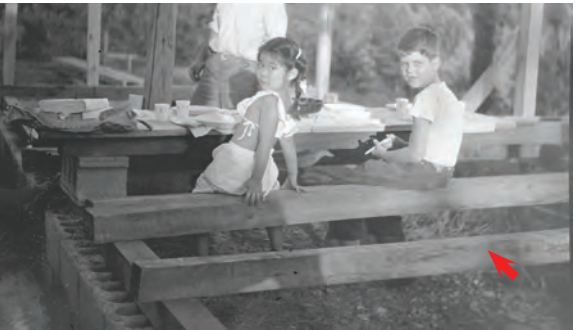
Figure 14.10 | A view looking east of the floor joists resting on the summer beam positioned on the concrete blocks of the crawl space during the construction, ca. August 1947 (Source: Nakashima Foundation for Peace).
